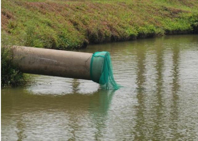
Figure 3: Protection of inlet pipe with a mosquito net bag
